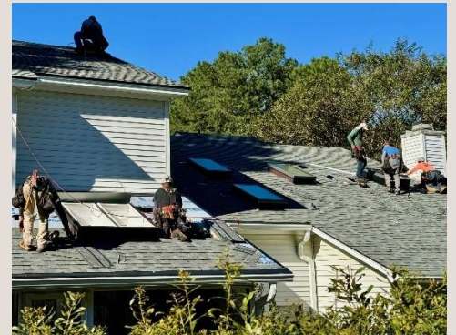
New roofing installed at Sycamore Close photo curtesy of Tony Daniels
