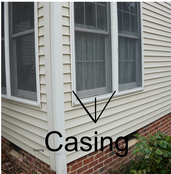
Window casings are the "trim" around the outside of a window
