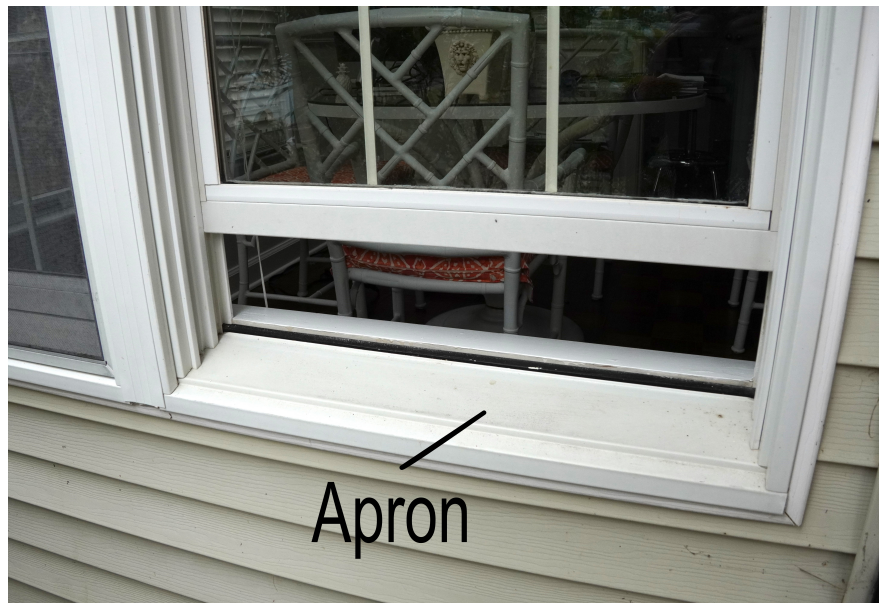
An apron is the sloping outside area behind the inside sill
